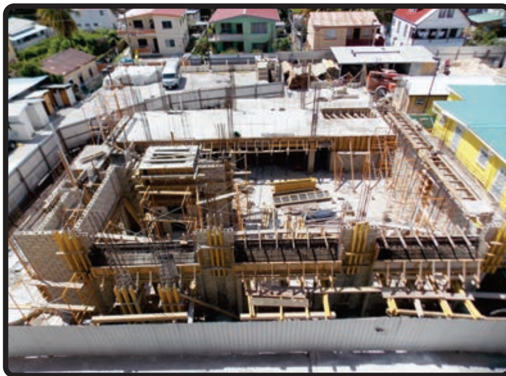
HRCU's building expansion well underway at #1 Hydes Lane
